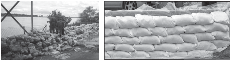
Figure 2 Incorrect and correct construction of provisional embankment
