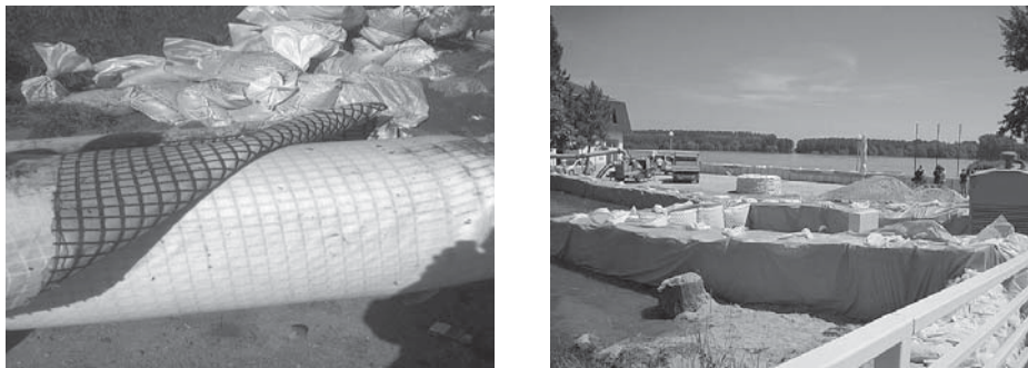
Figure 3 Impermeable foil for ensuring primary embankment and box barriers used for constructing embankments
