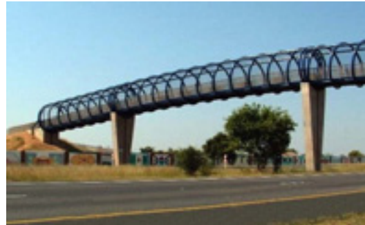
Figure 3: N1 Freeway Pedestrian Bridge
