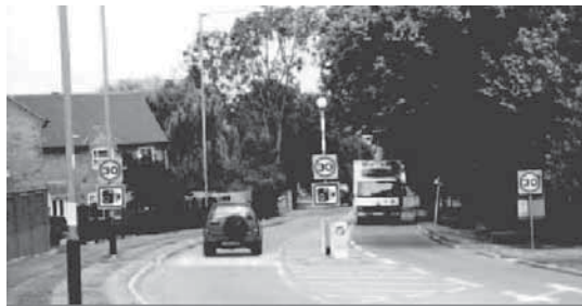
Fig.8: Directing fields in the central part and surface of part of the carriageway painted in different color (on the left side)
